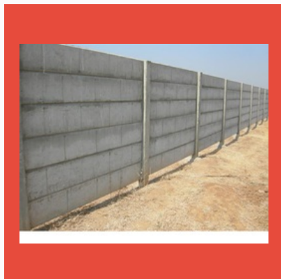
RCC Compound Boundary Wall
